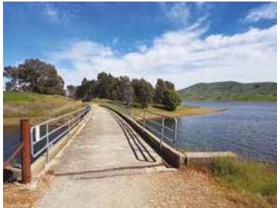
Sandy Creek Bridge
